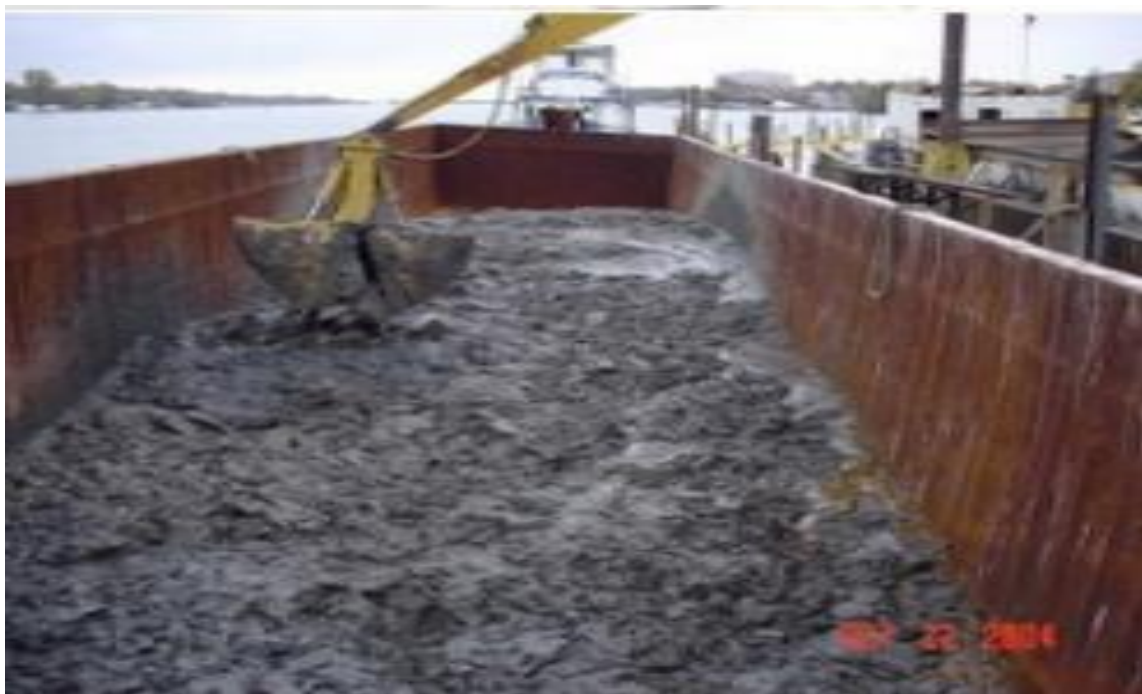
Figure 6- Storage dredged material in barge
