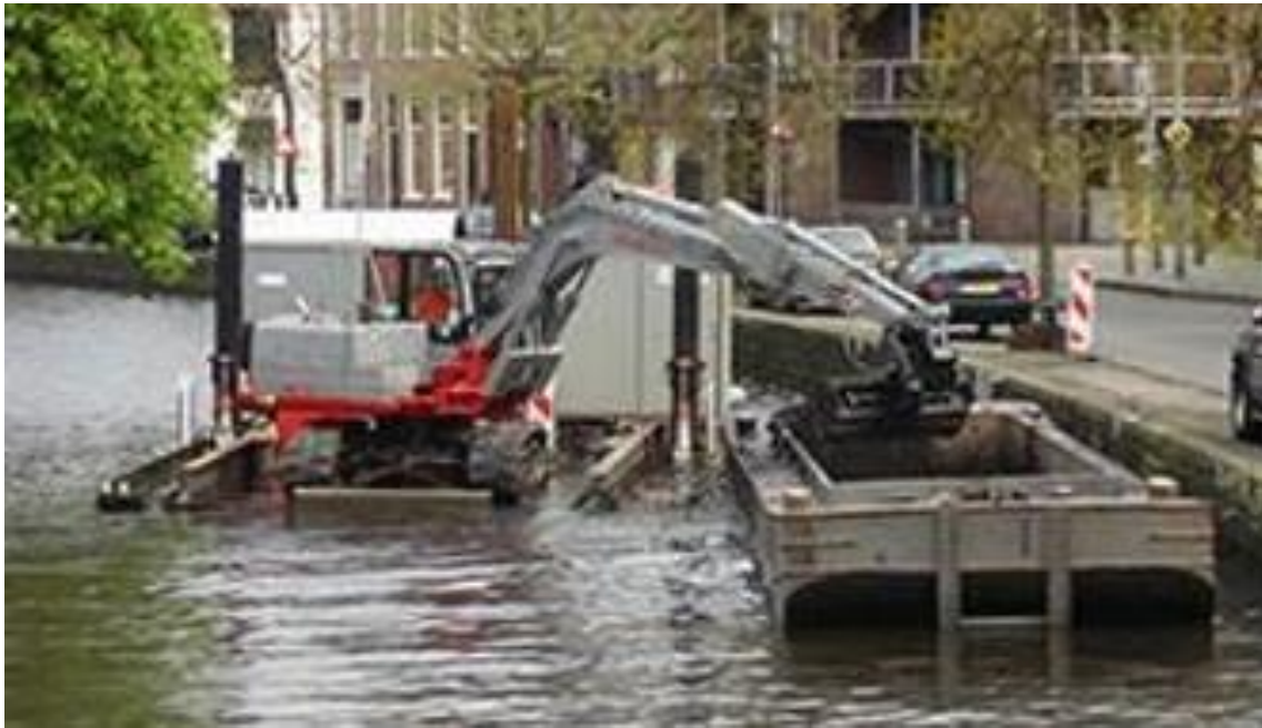
Figure 5- Excavator on a pontoon loading a barge
