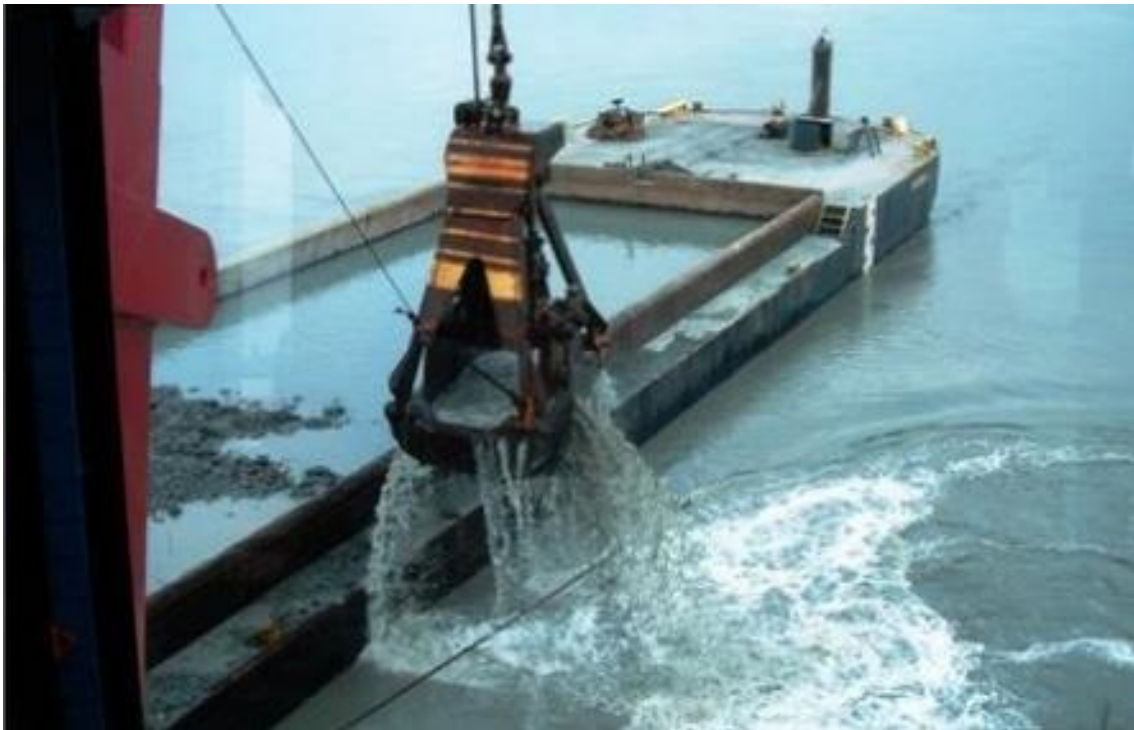
Figure 7- Dredged material being pulled out
