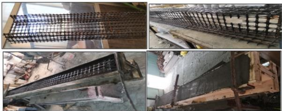
(B) Beams reinforced with tensor mesh.
