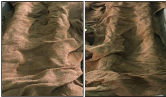
Figure 5: Curing of the beams with wet burlap.
