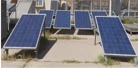
Figure 5- The installation of the 1.4 kW PV system
