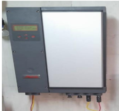
Figure 6- Central inverter for 1.4 kW PV system
