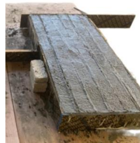
(c) After pouring.
