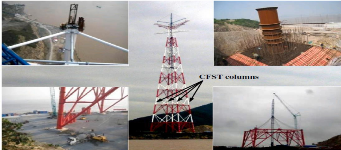
Figure 1- Uses of CFST columns
