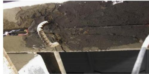
B) Epoxy-concrete interfacial de-bonding.
