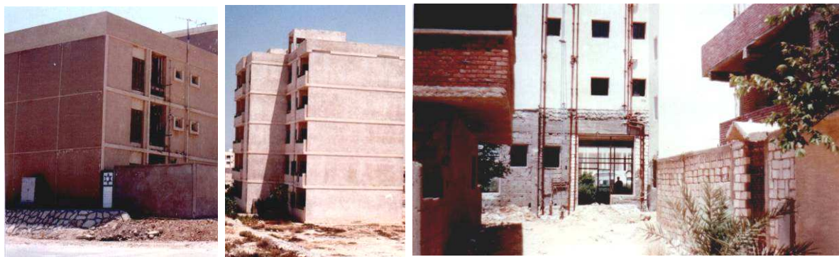
a. The tunnel system b. Different kinds of bricks used in building Fig. 2 The tunnel system and brick types used in building the houses in New Borg EL-Arab
